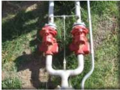
"GAS BOY" FUEL PRESSURE REGULATOR VALVES AND THERMAL RELIEF CIRCUIT
